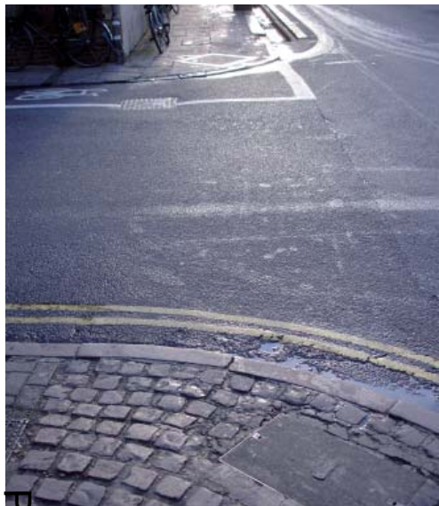
Granite setts instead of tactile paving (Trumpington Street)
