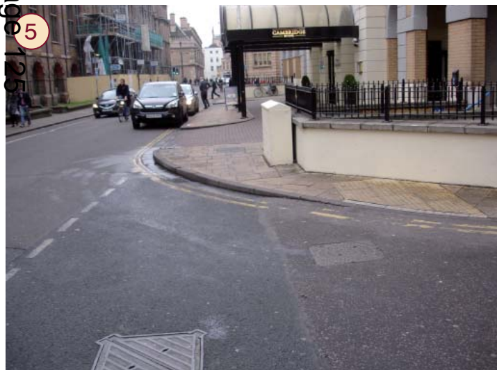
5 Tactile paving leads visually impaired into a low wall. Then need to cross two vehicle accesses with no dropped crossings or tactile paving
