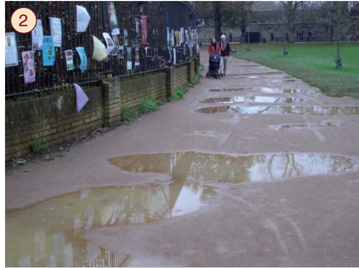
'Hoggin' path uneven and floods after rain
